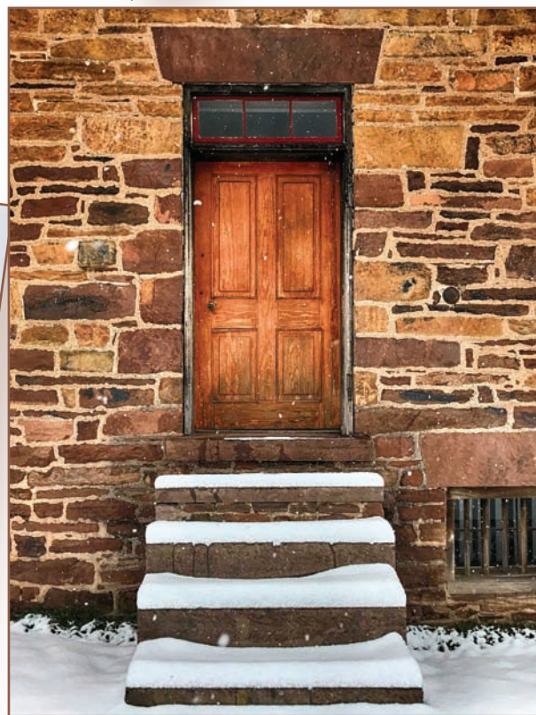
Stone House Entrance
