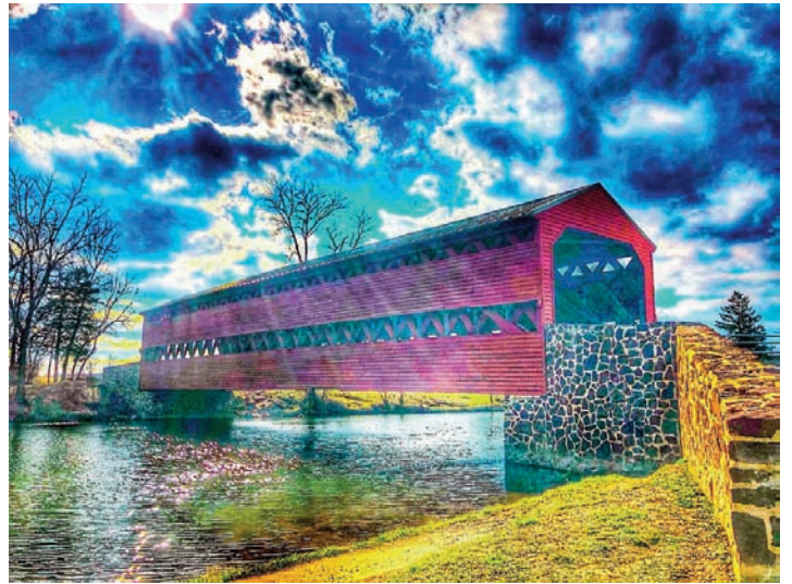
Sachs Bridge, which was used by both armies before and after the battle
